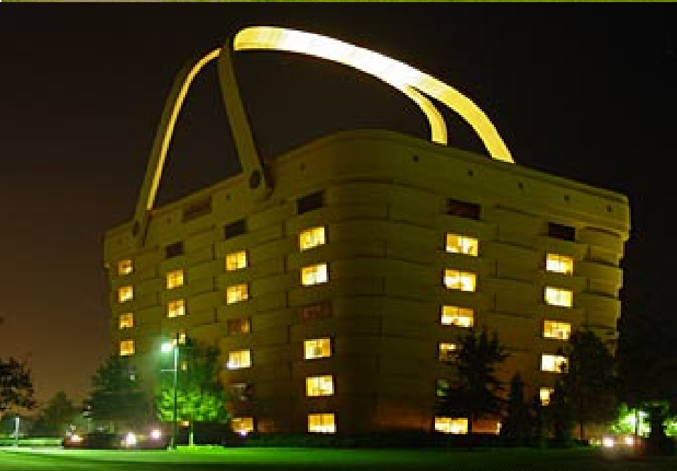
7-story building shaped like a basket is Longaberger's Home Office, Newark, Ohio.
